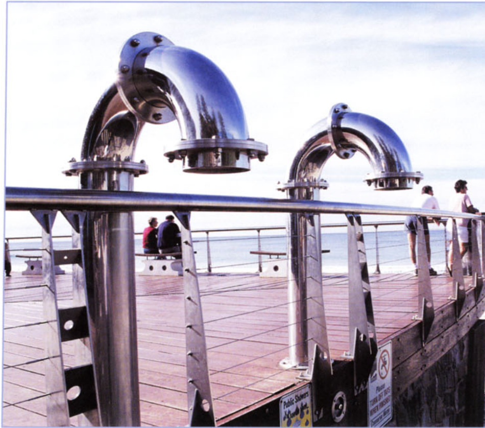
ABOVE: A successful stainless steel installation in a coastal application, with no tea staining.
